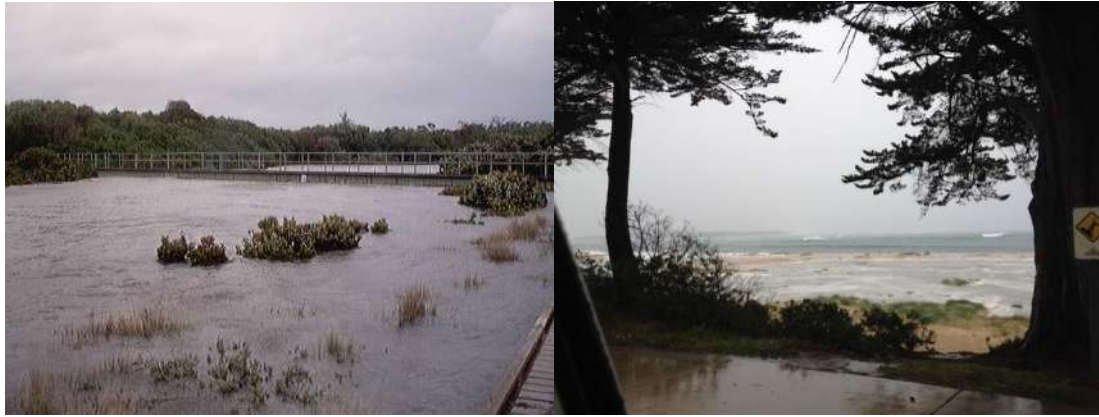
Figure 19: Photographs of the Screw Creek pedestrian bridge and from Surf Parade of the storm surge on 19 June 2004 (Courtesy of SGCS members).
