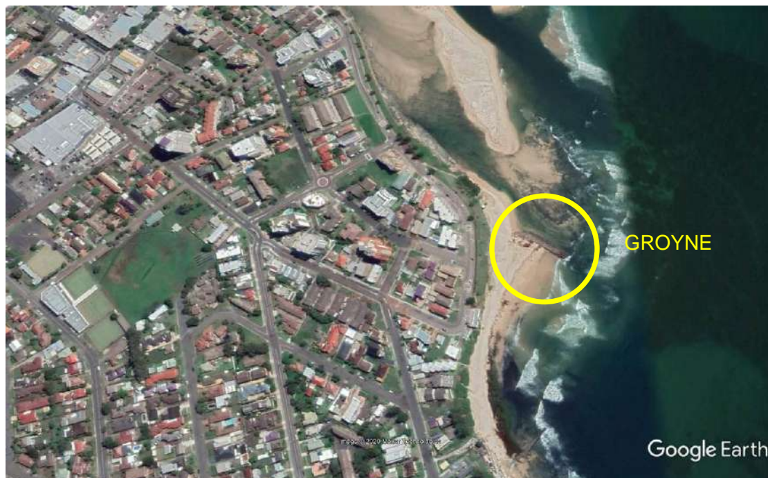
Figure 25: Groyne constructed at Tuggerah Lakes entrance to maintain the beach to the south
