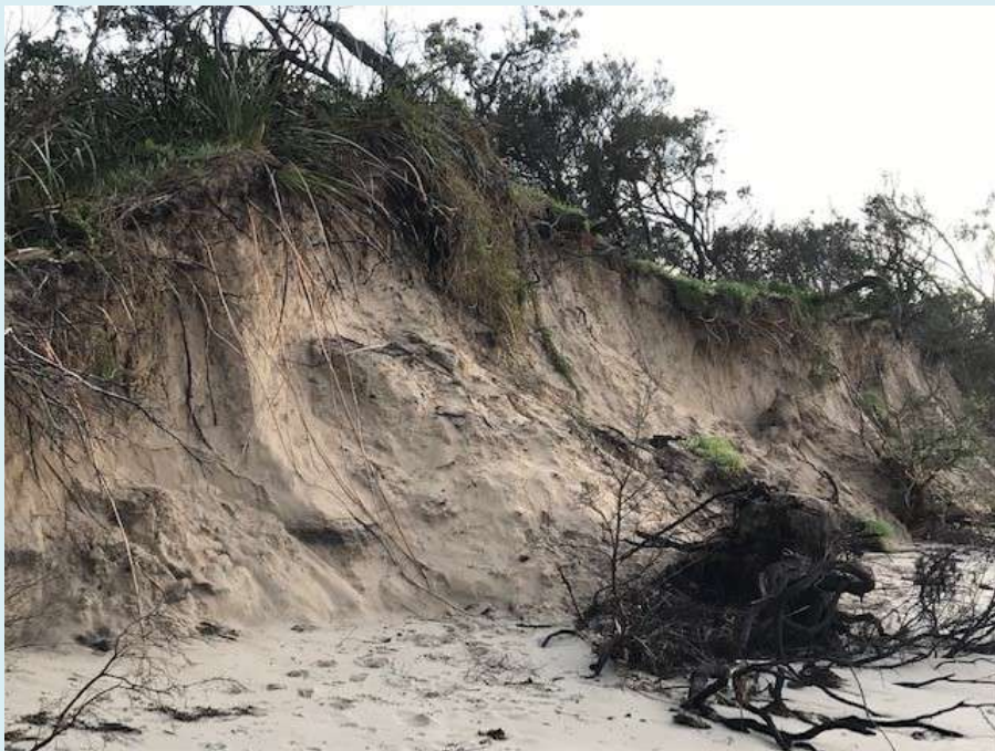
Coastline recession 50 metres west of CPR rock wall, 28 August 2020
