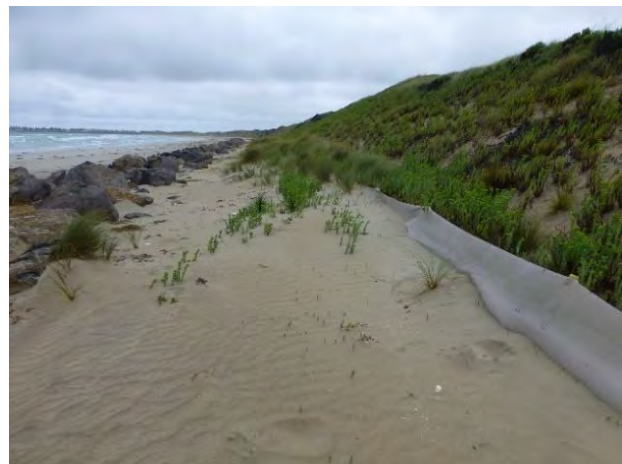
Fig. 37: Fence covered with geotextile material behind rock Wall, East Beach, Port Fairy
