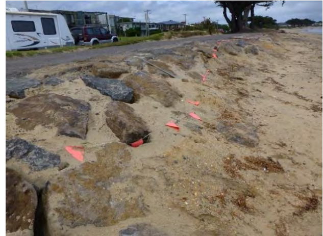
Fig. 49: Revetment works adjacent to Great Ocean Road, Apollo Bay
