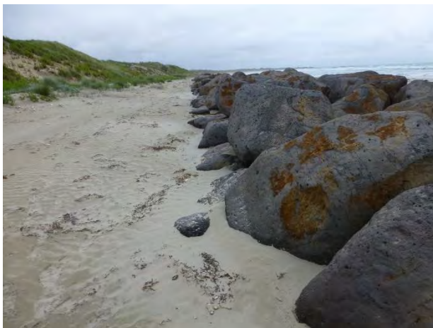
Fig. 36: Double layered rock wall, East Beach, Port Fairy
