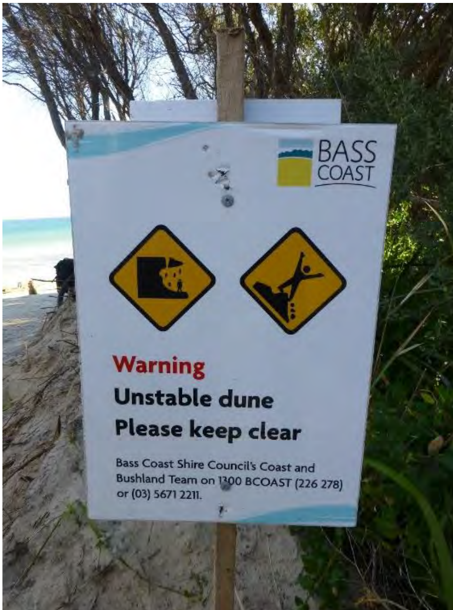
Fig. 55: Signage at Inverloch Surf Lifesaving Club indicating dune erosion hazard
