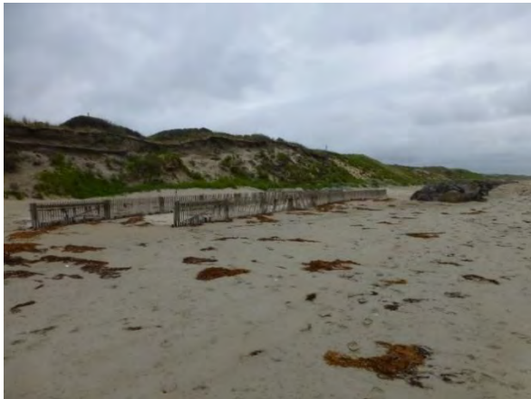
Fig. 38: Double trap sand fence at end of rock wall East Beach, Port Fairy
