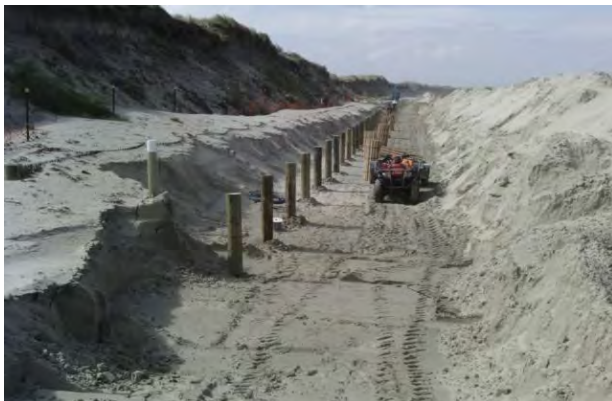
Fig. 40: Sand fence installation, East Beach, 2013 Source: Wattle & Wire 2018
