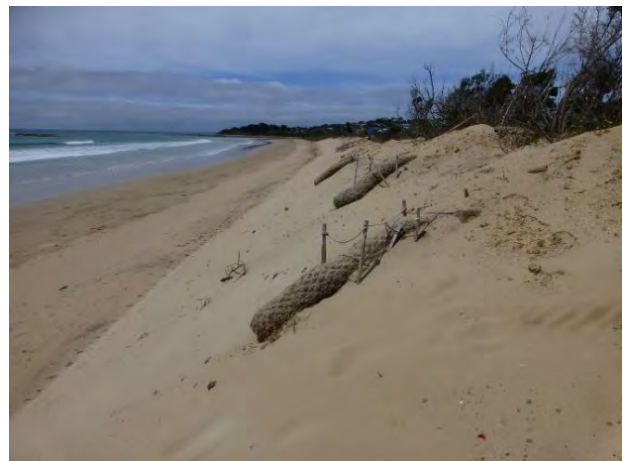
Fig. 45: Coir logs at Marengo Beach, Apollo Bay
